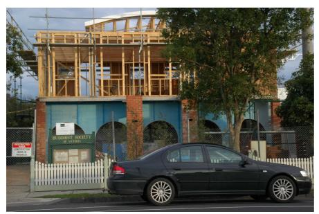
As can be seen, the frame is substantially complete – except the porches. By the time this newsletter is published, the roof should be completed.
